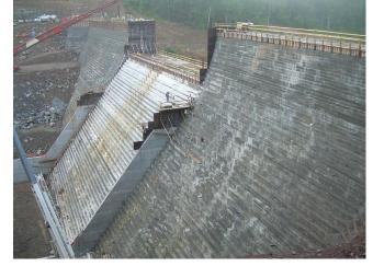
discharge, high turbulence levels, and intense flow aeration. Modern stepped spillways may have moderate to steep slopes and can accommodate large unit discharges. Because flow patterns of stepped spillways differ significantly from those on smooth chutes, designers must carefully analyze stepped chutes as their hydraulic design is far from trivial. An overview of the Workshop Program follows:
